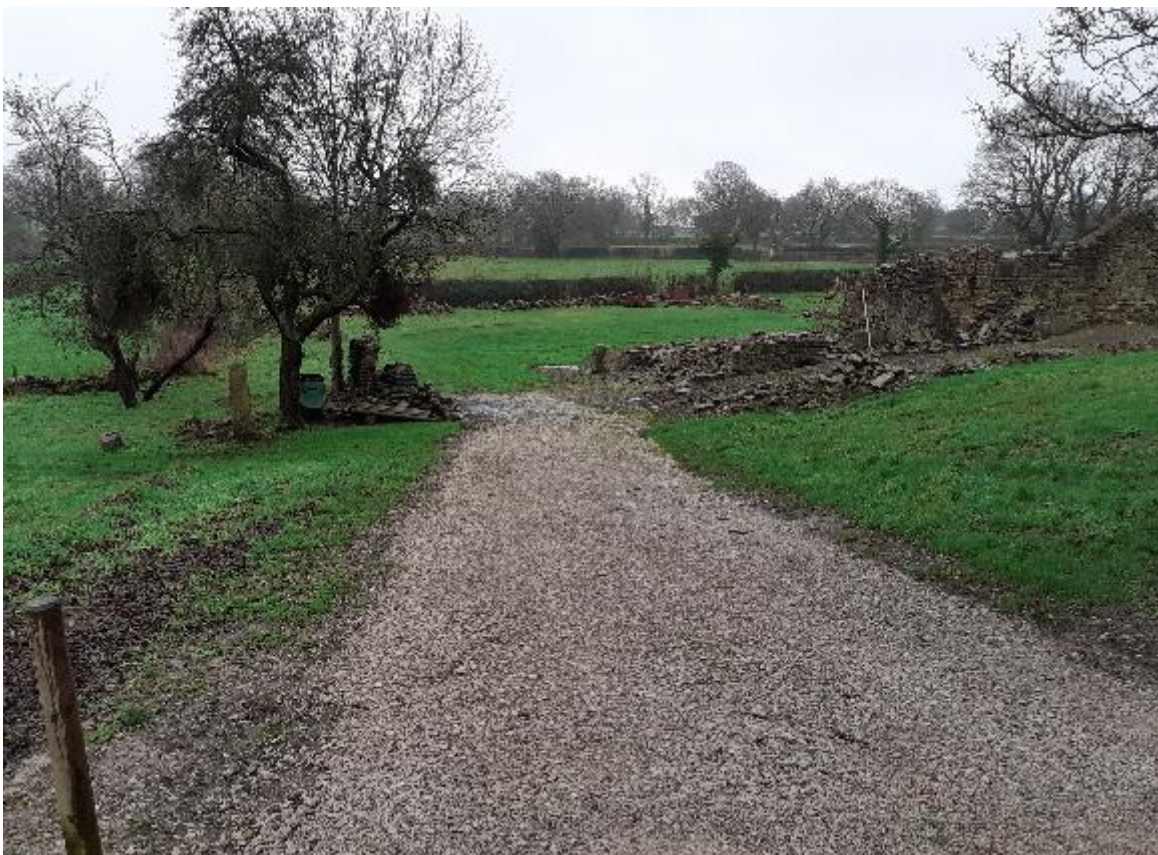
Figure 7: Site seen from site access (1)
